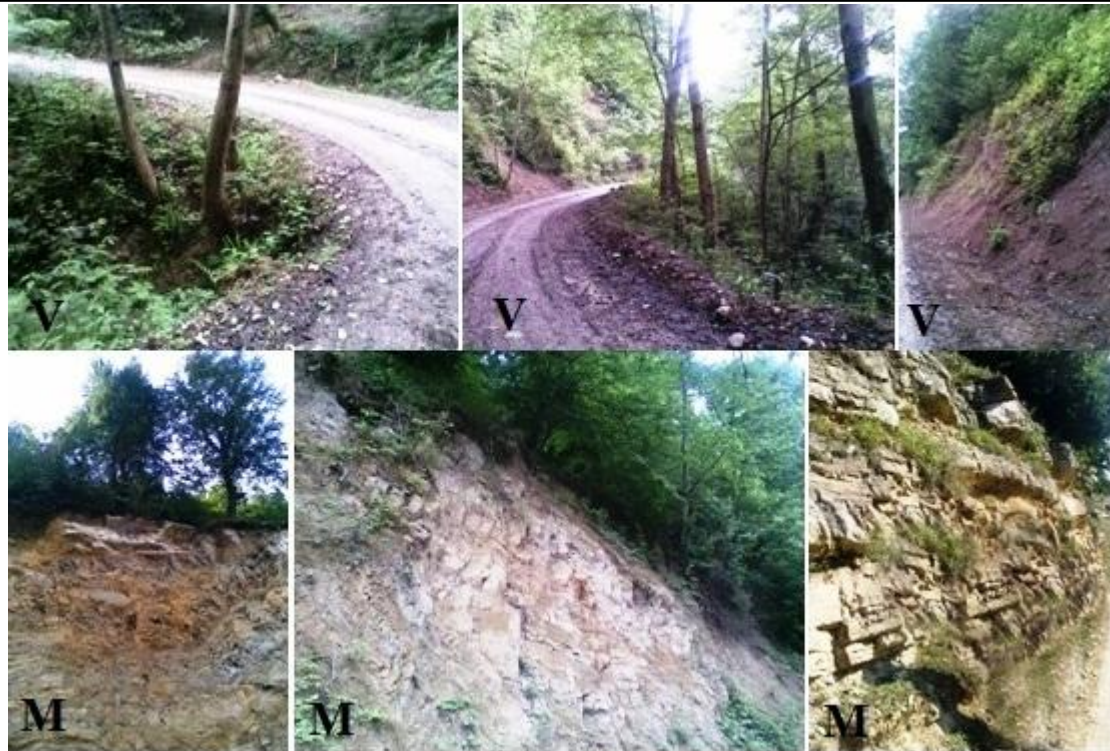
Figure 3: Real right of way in mountainous (M) and valley (V) forest roads
